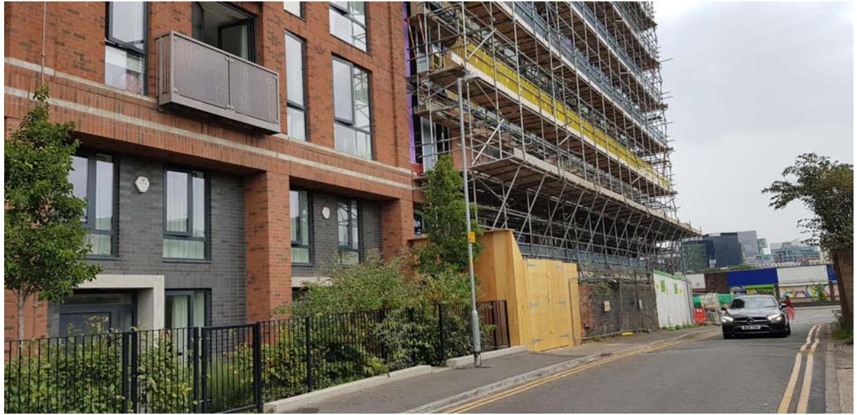
View (above) along Upper Wharf Street showing remains of the canal parapet wall
